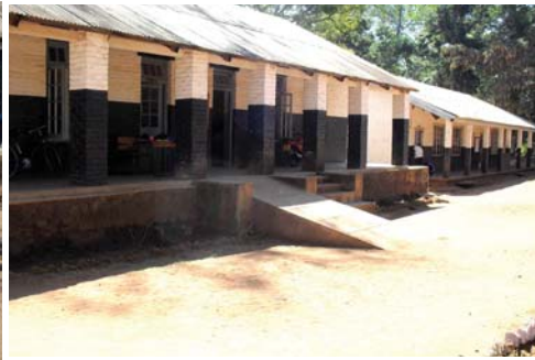
Pic 2. One of the ramps to improve access to classrooms.
