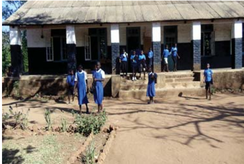
Pic 1. Domasi School steps before intervention.
